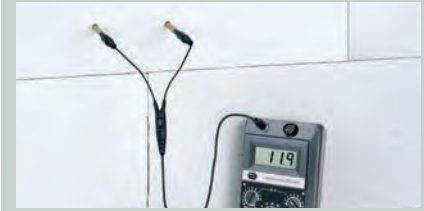
APPLICATION Measuring structural moisture using the RTU 600 unit and an M 21-100 deep measuring electrode pair
